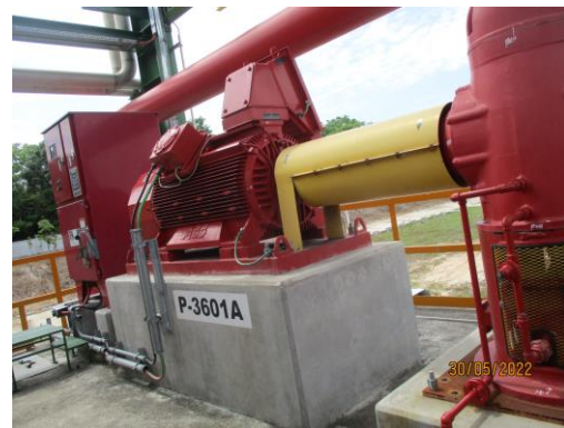
Electrical Driven Fire Water Pump
