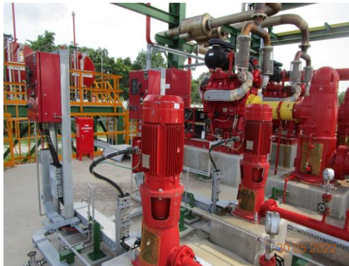
Electric Motor Driven Jockey Pumps
